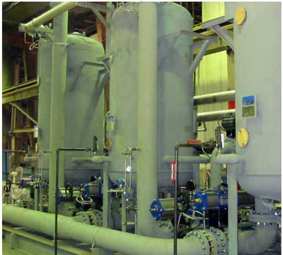
**Powdex three-vessel condensate polishing system**
